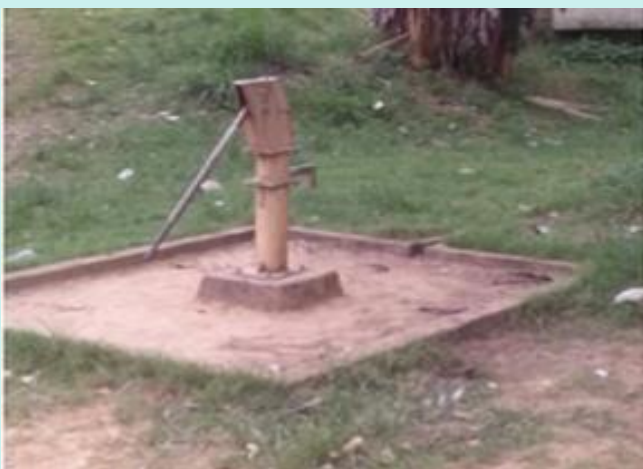
Fig. 5: Bore hole provided by a private stakeholder to a school which is now out of use
